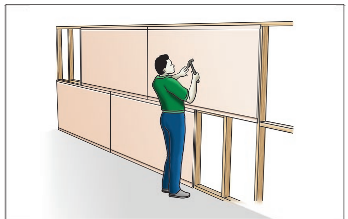
FIGURE 5 FIXING REMAINING SHEETS
